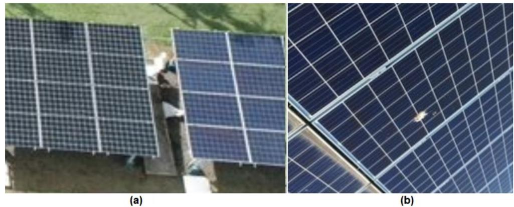
**Figure 1.** (a) PV-chain with partial shade due to a tree, (b) PV-chain with dirt due to a bird drop.
