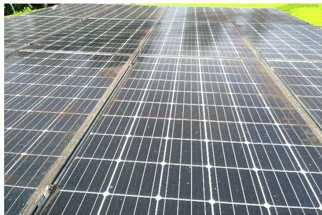
**Figure 2.** Monocrystalline PV module analyzed with the presence of natural non-uniform dirt.
