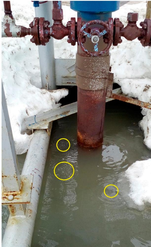
**Figure 13.** Gas liberations from permafrost around working well at Yamburg gas field (Yellow circles—locations of gas liberations, photo by N. R. Avetov).
