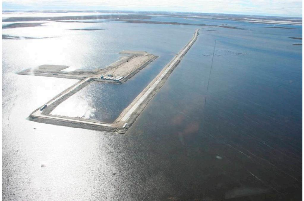
**Figure 9.** Springtime waterflooding around well cluster plot in the North of West Siberia (photo by A. P. Popov).
