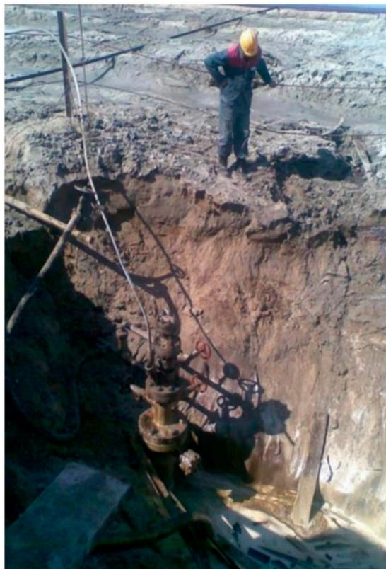
**Figure 12.** Surface subsidence and wellhead movement caused by permafrost thawing around gas production well (Zapolyarnoye gas field, West Siberia [9]).
