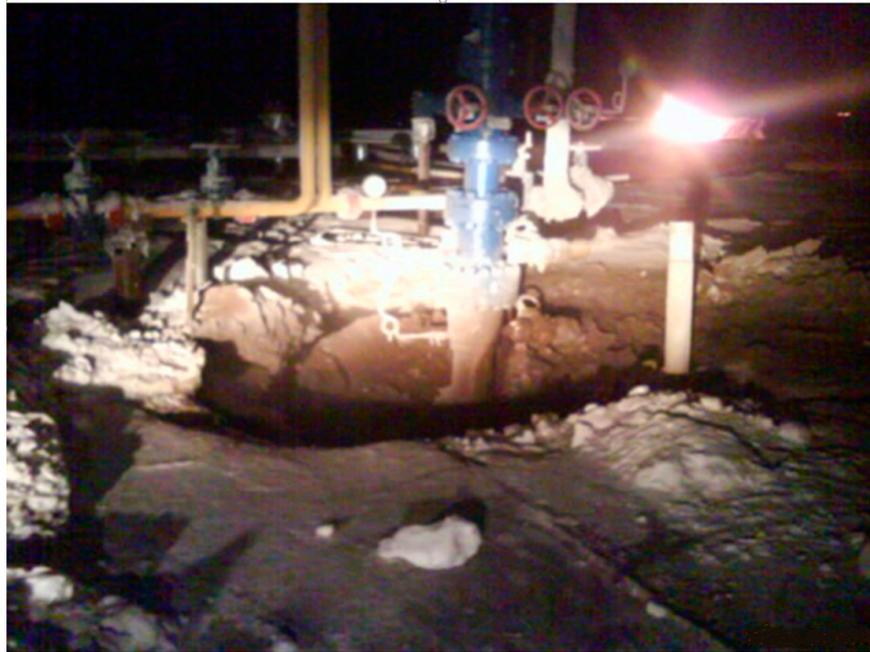
**Figure 11.** Typical spring well-site surface subsidence around working gas well [21].
