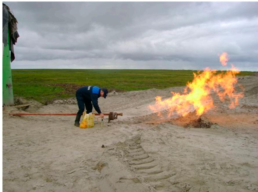
**Figure 14.** Permafrost and hydrate-stability zone degassing before production well drilling [29].
