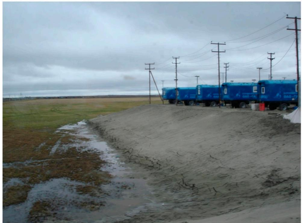
**Figure 8.** Sand pillow for drilling rig and well cluster in the North of West Siberia [29].
