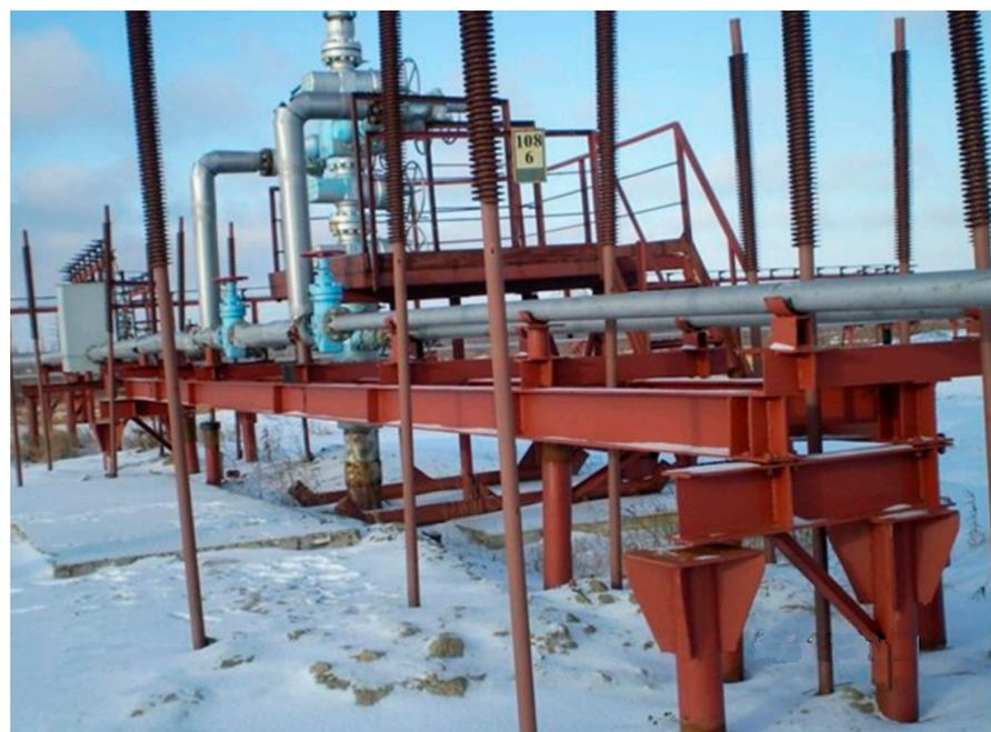
**Figure 16.** Wellhead support with seasonal cooling devices (SCDs) around piles keeping ground frozen all year round [21].
