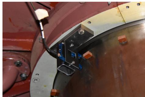
**Figure A12.** Upper sensor installation below the lower generator bearing.
