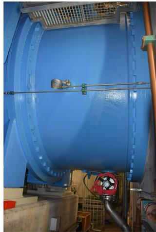
**Figure A2.** Position of the spiral case pressure sensor.
