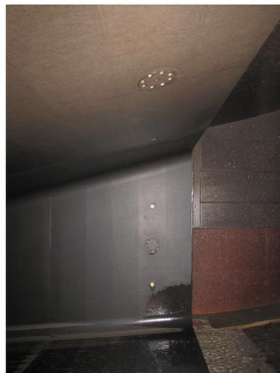
**Figure A8.** Position static pressure measurement taps at the end of the draft tube  $p_{DT}$ .
