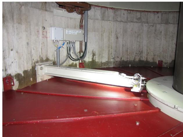
**Figure A4.** Regular speed sensor.
