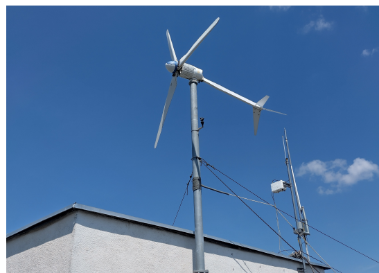
Figure 1. A wind turbine equipped with 700 W PMSG.
