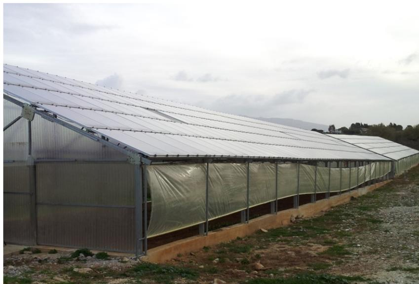
For the realization of the PV system multicrystalline silicon panels have been used, a less expensive material than monocrystalline ones, because of the simpler manufacturing process required, even if slightly less efficient [54].
