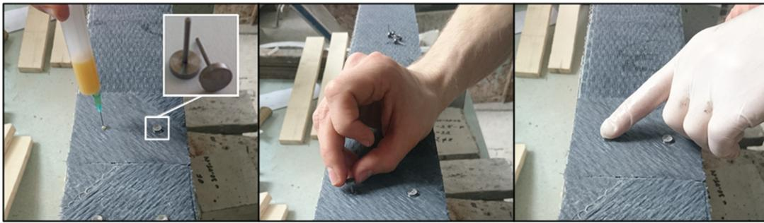
Figure 11. Installation of steel pins.
