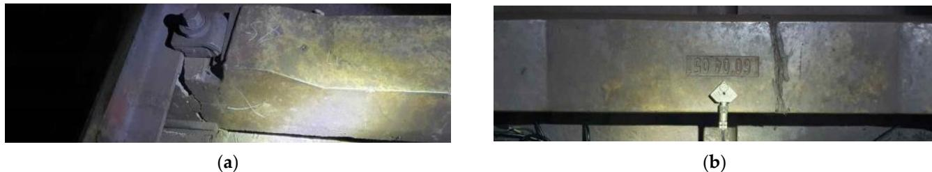
**Figure 12.** Damage of concrete sleepers. (a) Bottom of the rail; (b) center of concrete sleeper.
