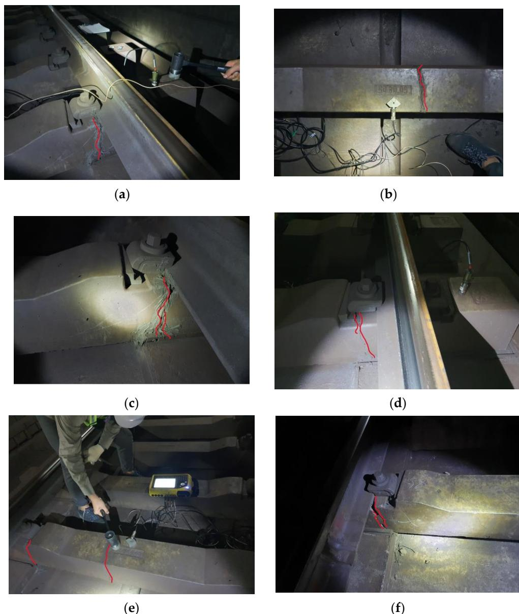
**Figure 1.** Visual inspection of concrete sleepers. (a) Crack #1 (rail seat); (b) Crack #1 (center); (c) Crack #2 (rail seat); (d) Crack #2 (rail seat); (e) Crack #3 (rail seat, center); (f) Crack #3 (rail seat).
