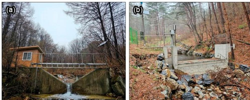
**Figure 2.** Views of stream gauging stations in (a) C19 and (b) C27 among observed forested catchments (C1–C39). 120° V-notch and rectangular sharp-crested weirs were installed in C19 and C27.
