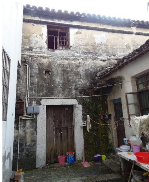
**Figure 6.** A Tianjing-style courtyard built in the Qing Dynasty that now belongs to three families. The three-story concrete brick architecture on the left side was built in 2000 after the original house was demolished; the single-story house on the right side was also built after the original house was demolished, but the completion time is unknown; only the traditional brick wood architecture in the middle was preserved, but it was uninhabited. (Photograph by Fengyi Ji.).
