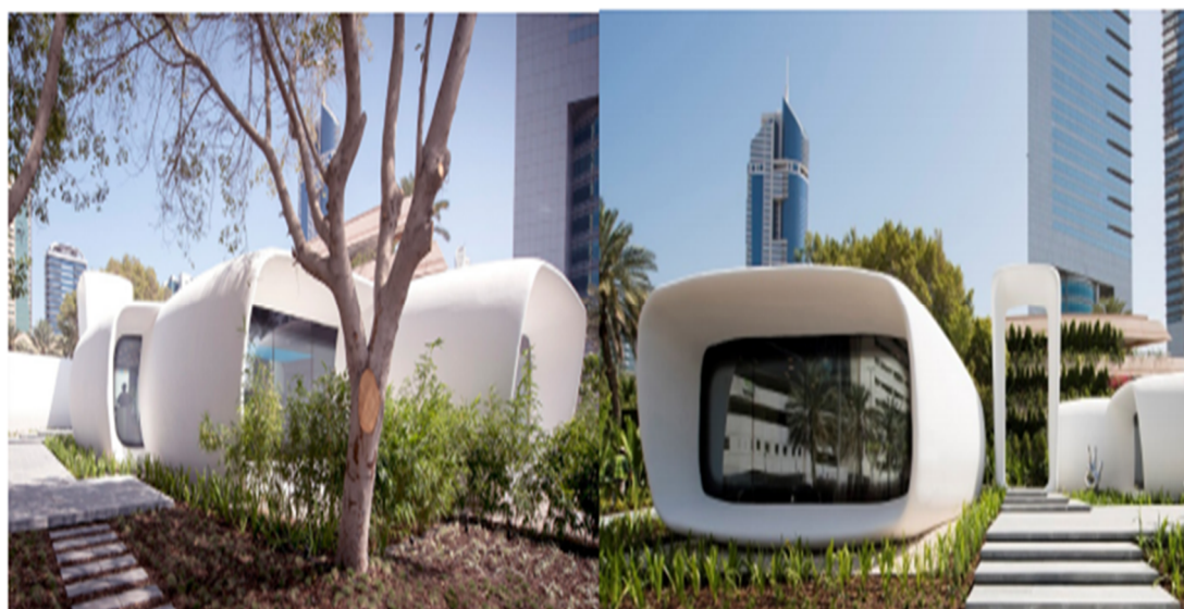
Figure 4. Front view and side view of “Office of the Future” in Dubai, manufactured by 3D printing technology [11].
