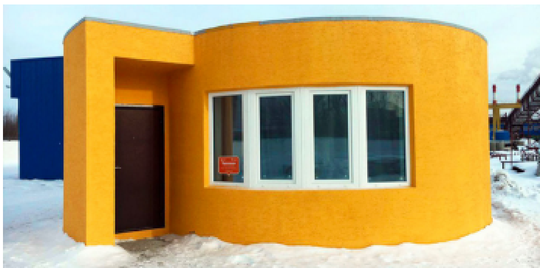
Figure 6. The 3D-printed building “Apis Cor House” was constructed in Russia [11].
