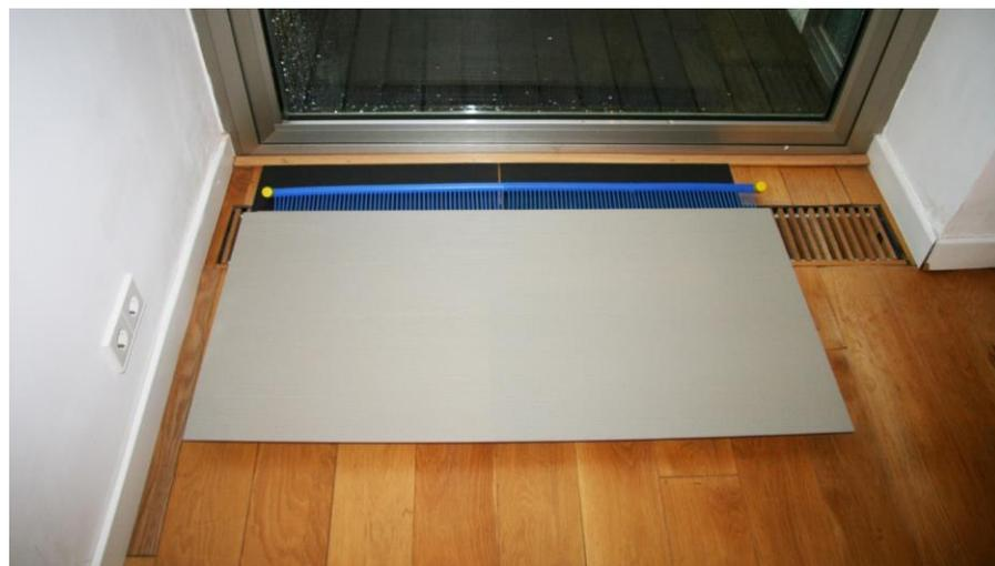
**Figure 4.** Possible on-site application of the TCP panels in its different layers.
