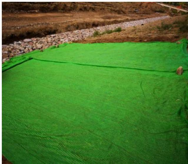
**Figure 9.** Slope surface covered with blanket after seeding.
