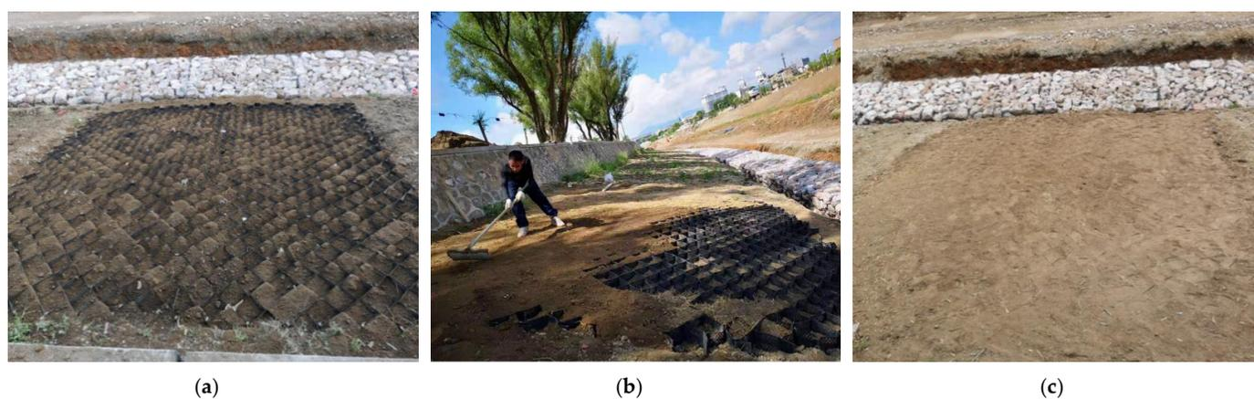
**Figure 8.** Infilling of the top soil: (a) bottom 10 cm of bare soil; (b) infilling from the crest to the toe; (c) the finished slope after treatment.
