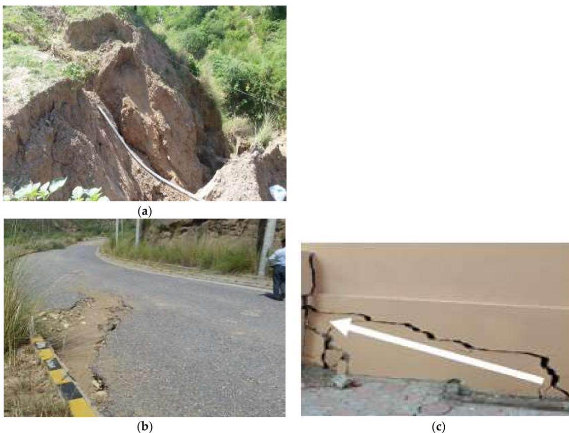
**Figure 1.** Serviceability issues at the study site: (a) Shallow slides; (b) Pavement defects; and (c) Building crack.
