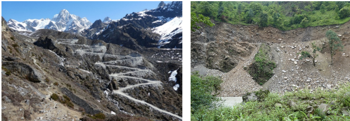
Figure 3. (Left) Road construction in 2019 over the Tiptola Pass (5095 m) to Tibet. (Right) Landslides from new road construction across from Japantar in 2022 (photographs by A. Byers).
