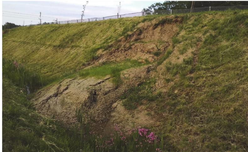
**Figure 2.** Example of a road landslide in the Polish Carpathian region.
