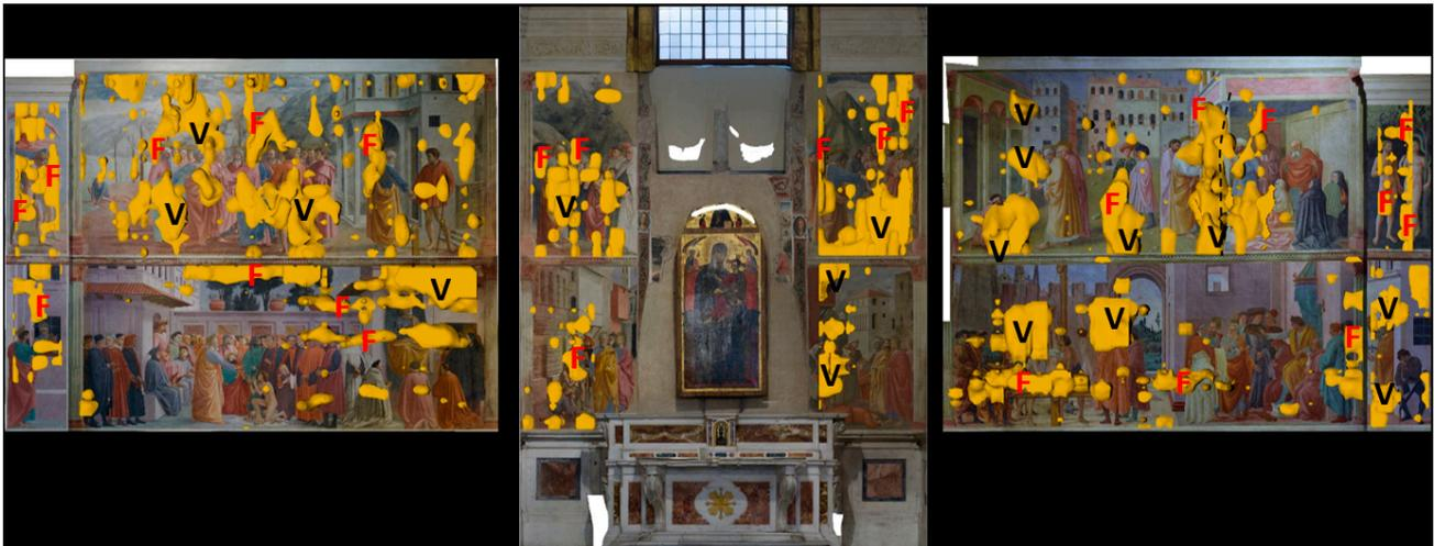
Figure 10. 900 MHz antenna: anomalies found (V: void spaces; F: fractures).
