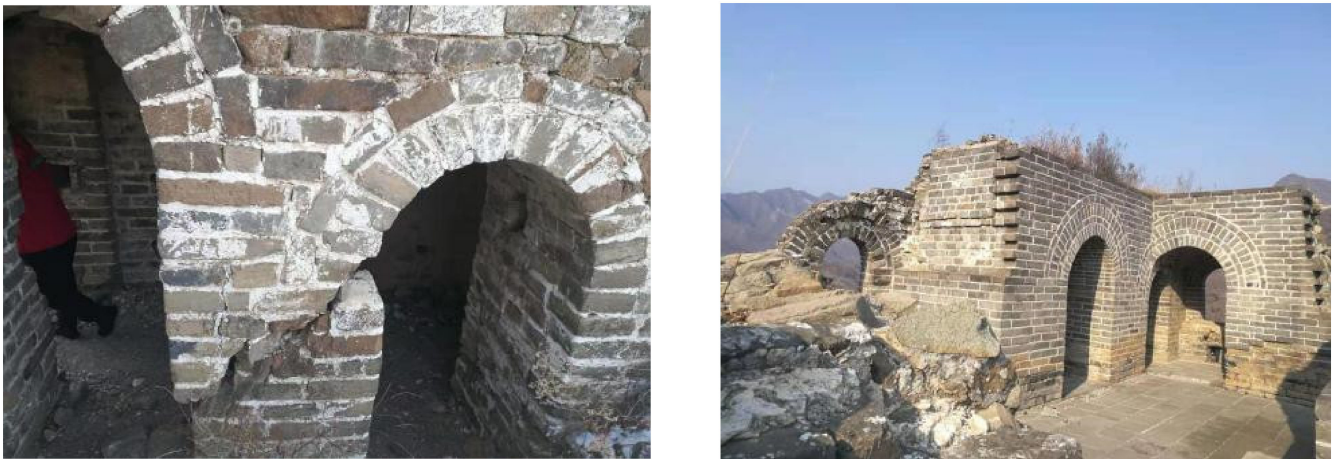
Figure 9. Deformation (left) and collapse (right) of the Great Wall.
