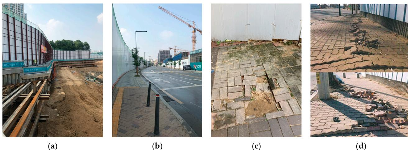
**Figure 1.** (a) Supporting wall and safety fence standing at an excavation site; (b) block pavement for pedestrians adjacent to the safety fence outside the excavation site; (c) example of misaligned blocks adjacent to the safety fence; (d) example of severe distortion in the block pavement.
