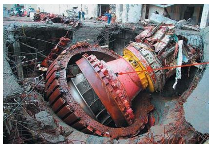
Figure 16. Pushing the multi-ton turbine assembly up during the Sayano-Shushenskaya HPP accident on August 17 2009.
