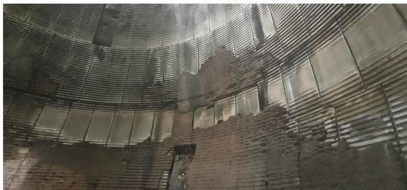
**Figure 1.** Slag crust adhered to the hot surface of the copper stove of the blast furnace.
