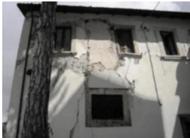
**Figure 1.** Damage concentrated at the irregularities on masonry buildings [28].
