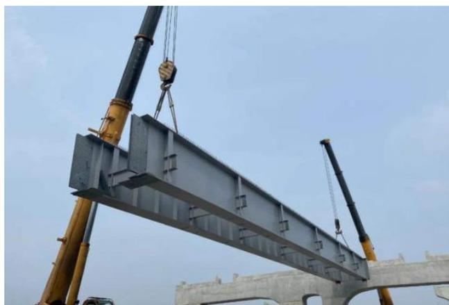
**Figure 1.** Steel plate girder in long-span structures.
