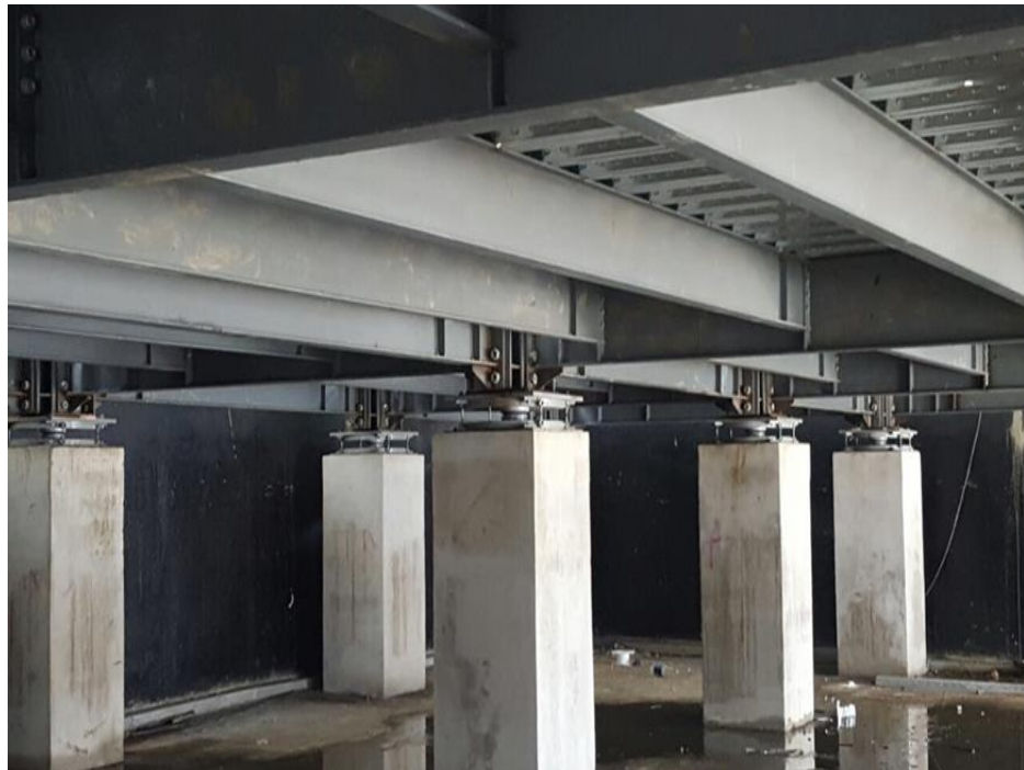
Figure 16. Dangerous EN15129 isolators installed on columns in a hospital in Ecuador.
