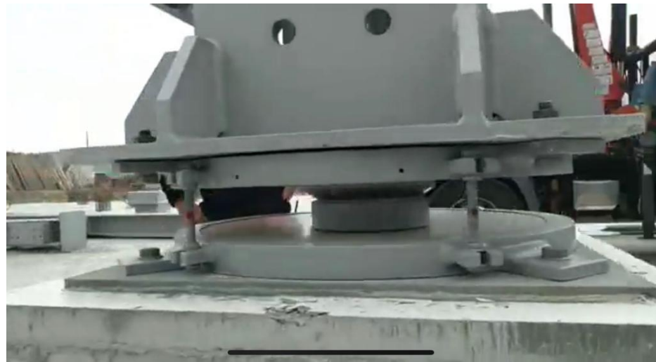
Figure 15. Dangerous EN15129 essentially flat isolator installed in a hospital in Ecuador.
