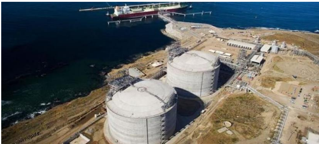
Figure 7. LNG Tanks, Mexico, 100% Functional after 2022 M7.6 Earthquake.
