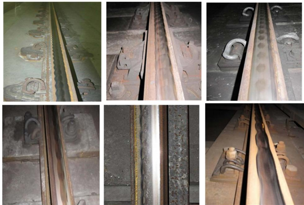
**Figure 11.** Rail corrugated in a resilient fastener section.
