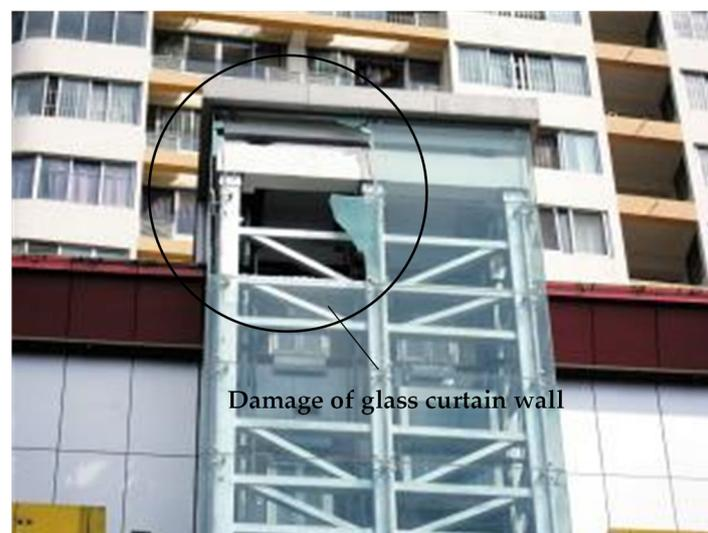
**Figure 2.** Damage to a glass curtain wall around the installed elevator shaft [45].
