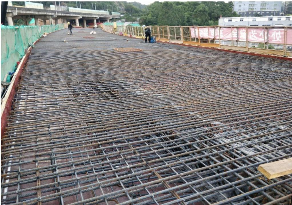
**Figure 1.** Rebar of the bridge deck slab.
