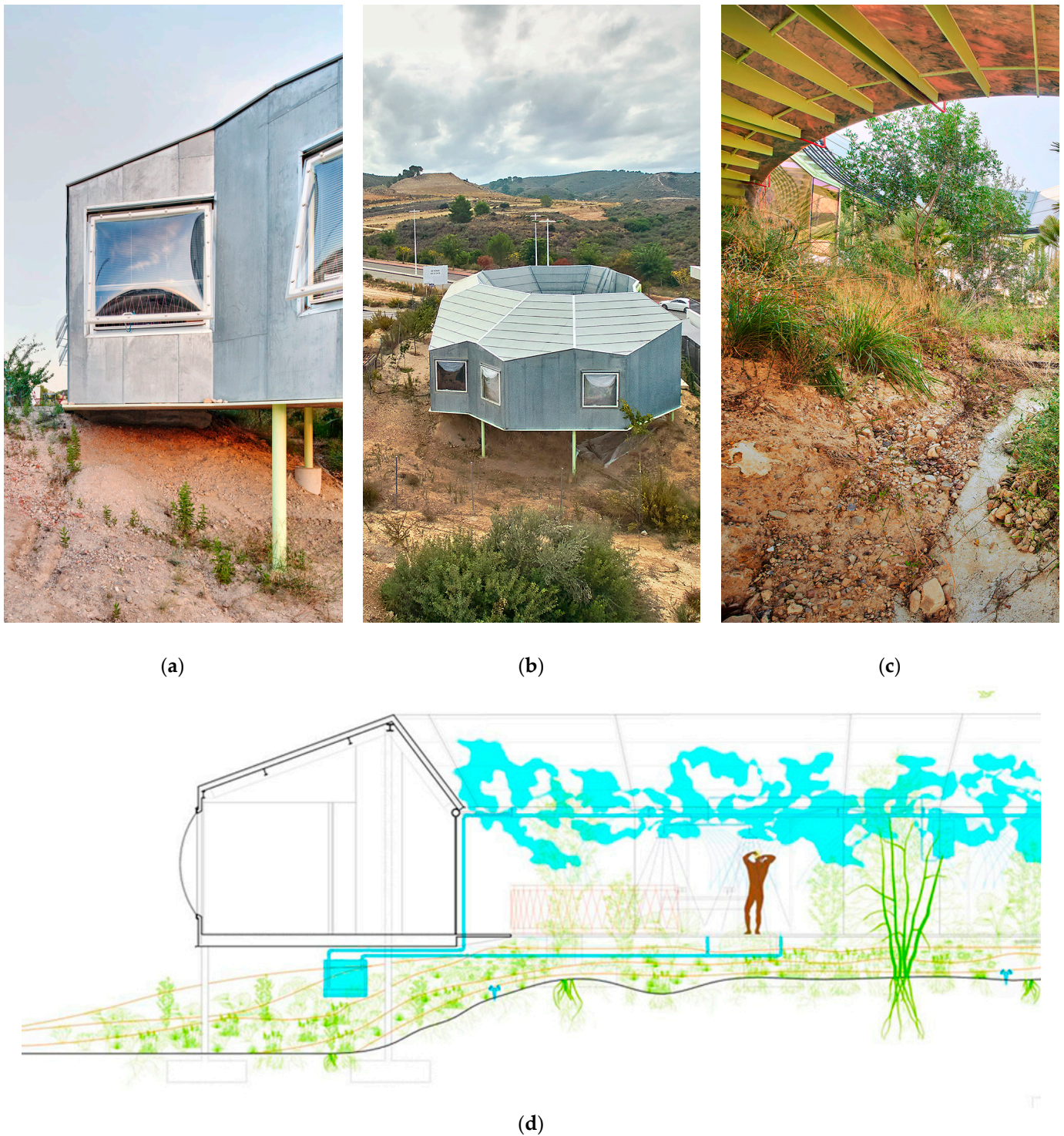
Figure 6. The Rambla Climate-House. Murcia, Spain. (A. Jaque and M. Mesa, 2022 [40]). (a) Detail of the rooting. (b) Aerial view. The house is built on stilts that rise from the ground (c) The house is organized around this elliptical void. The natural topography of the land is preserved. (d) Section (Fragment). Photography: José Hevia. Drawings: A. Jaque and M. Mesa. Images and drawings compiled by the authors Source: < https://officeforpoliticalinnovation.com/work/marblelous-crowned-house/ > (accessed on 18 February 2024).
