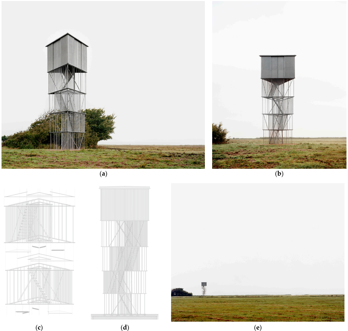
Figure 7. Tipperne Bird Sanctuary. Ringkøbing. Denmark (Johansen Skovsted Arkitekter, 2017 [43]). (a,b) The building is imagined as free-standing object in the landscape. (c) Exploded axonometric drawing (d) Section. The structural system is designed as a structure that expands as it grows, allowing for a small footprint on the ground. (e) View of the bird watching tower. Photography: Rasmus Norlander. Drawings: Johansen Skovsted Arkitekter. Images and drawings compiled by the authors. Source: https://www.archdaily.com/883075/tipperne-bird-sanctuary-johansen-skovsted-arkitekter (accessed on 18 February 2024).
