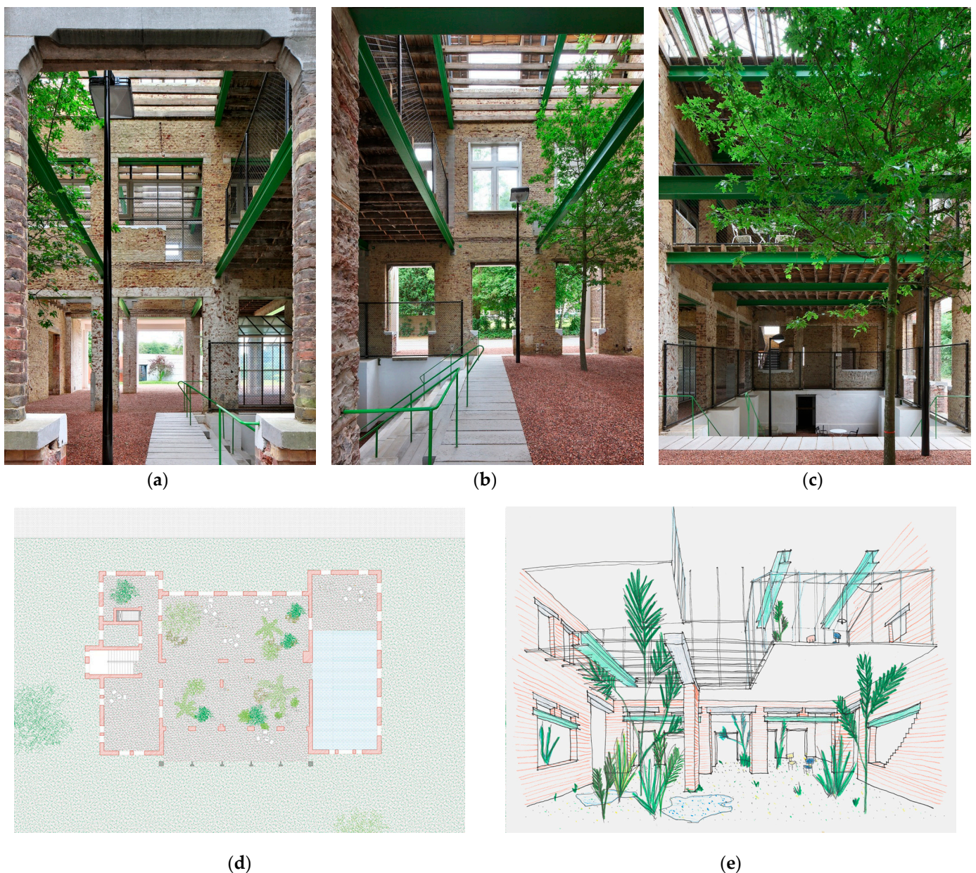
Figure 12. PC Caritas, Melle, Belgium (De Vylder Vinck Taillieu, 2019 [57]). (a–c) A new ground penetrates the existing building. This operation rehabilitates and converts the old space into an experimental public place where the boundaries between inside and outside are blurred. (d) Ground plan, (e) sketch. Photography: Filip Dujardin. Drawings: De Vylder Vinck Taillieu. Images compiled by the authors. Source: https://www.archdaily.com/871034/pc-caritas-architecten-de-vylder-vinck-taillieu (accessed on 18 February 2024).
