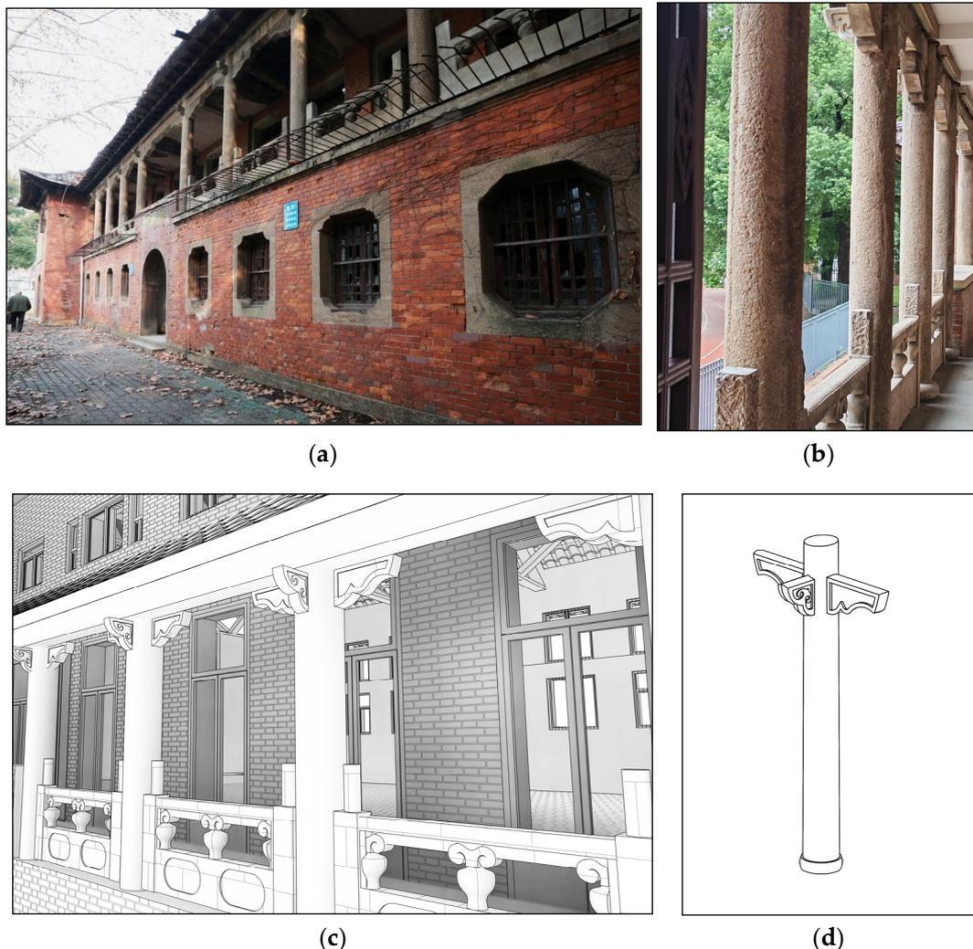
**Figure 16.** Component virtual repair (source: author). (a) Second-floor corridor of building. (b) Detailed pathologies of column members. (c) Virtually restored colonnade. (d) Virtually restored column family.
