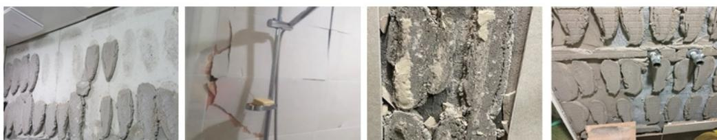
**Figure 1.** Types of bathroom wall tile defects.
