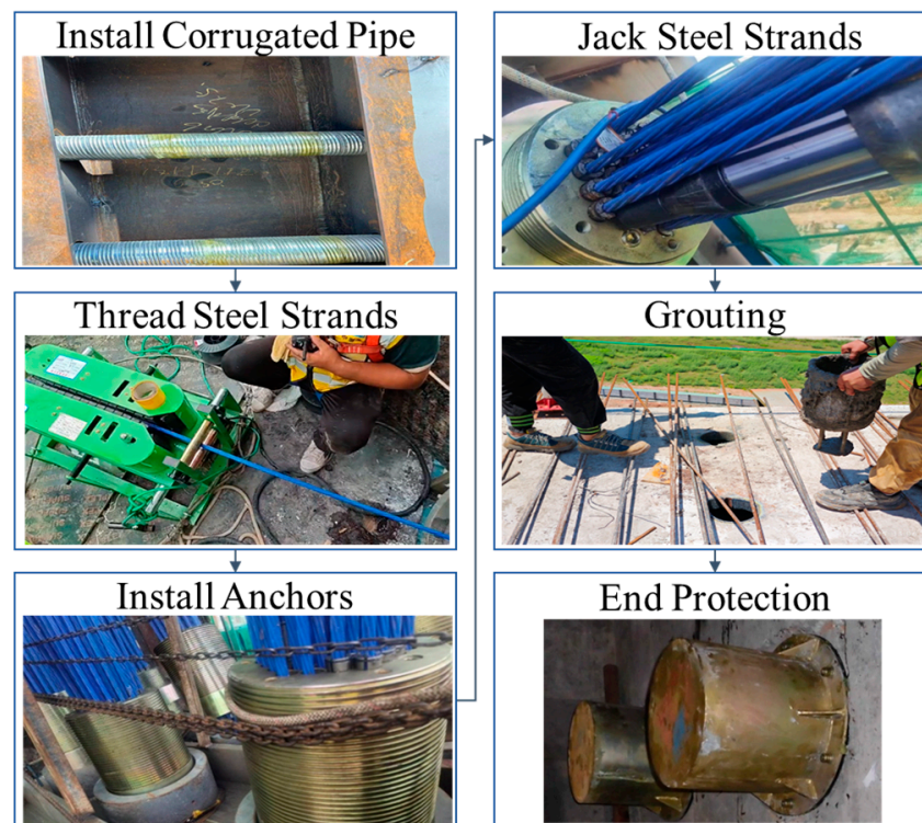
Figure 11. Prestressed construction steps.
