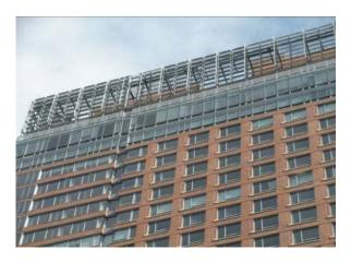
Figure 8. The Riverhouse dynamic PV system [28].
