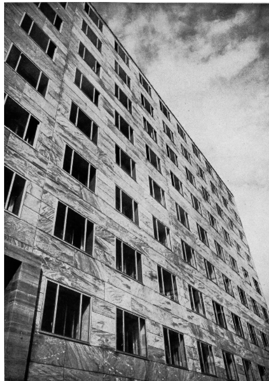
Figure 20. Montecatini office building by Gio Ponti. Milan (1936–1938). Side elevation. Cladding in cipollino apuano marble. Double Anticorodal frames. Photo from ( Diotallevi and Marescotti 1939 , p. 113).
