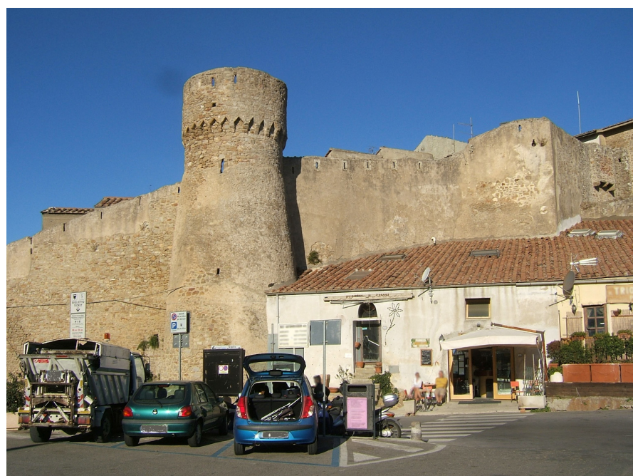
Figure 11. Giglio Castello: the walls of the 16th century, built with granite ashlar.
