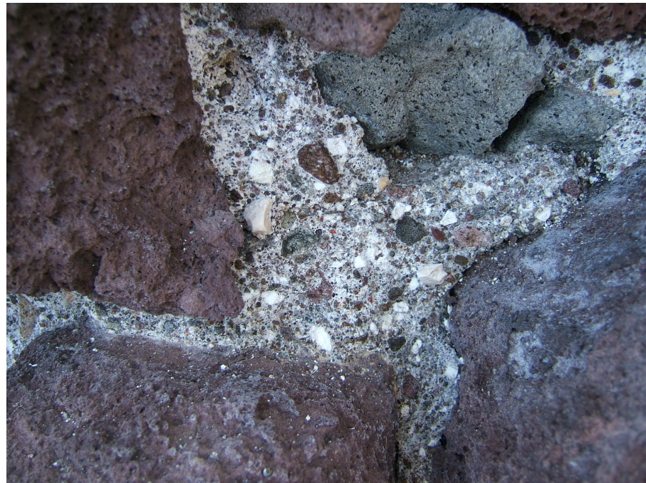
Figure 6. The high number of lumps in the bedding mortars of the Zenòbito Tower may indicate the technique of the hot lime in the realisation of mortars.
