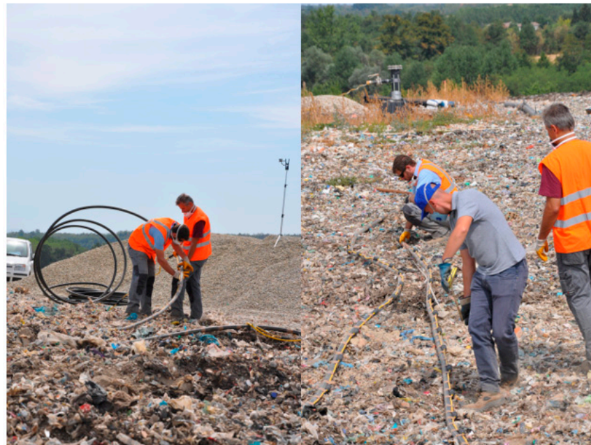
Figure 5. Phases of preparation and installation of the electrodes for borehole and cross-hole monitoring of electrical resistivity. The graphite electrodes are installed on the external side of the HDPE tube of the piezometers.
