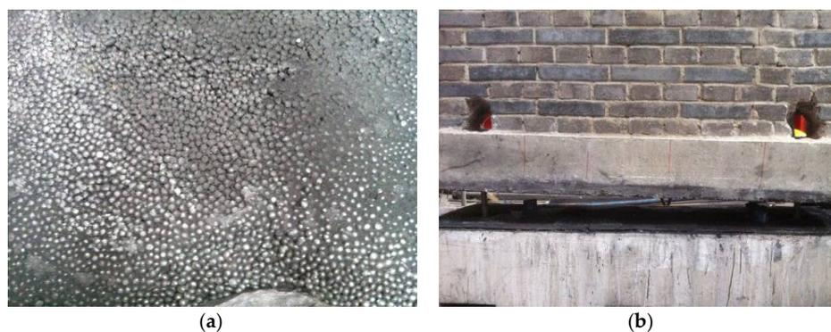
**Figure 8.** MG isolator: (a) MG mixture; (b) MG isolator in place.
