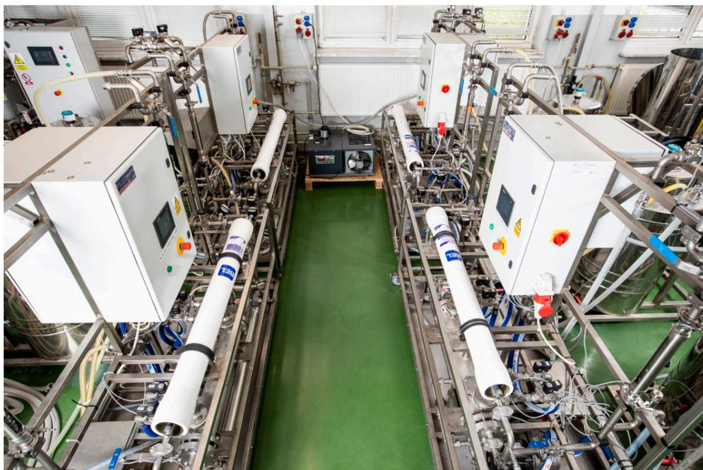
**Figure 1.** Integrated membrane system for industrial wastewater treatment.
