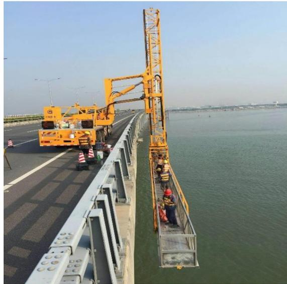
**Figure 1.** Manual bridge crack detection.
