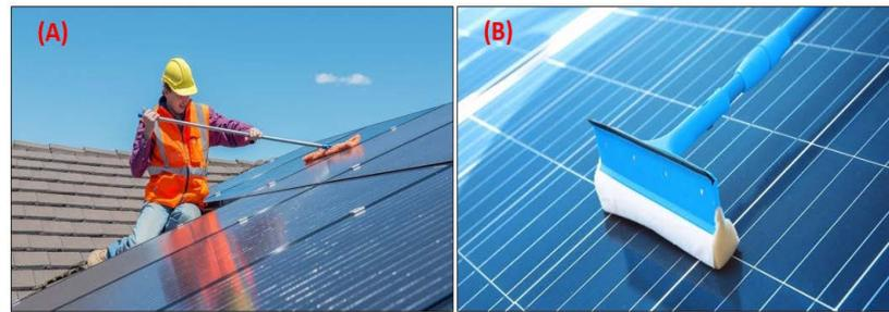
**Figure 8.** Manual cleaning process of the PV panels. (A) Using a soft brush with distilled water and dish soap, (B) using a soft brush.
