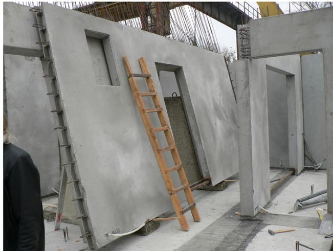
**Figure 10.** View of reinforced concrete panels with integrated ATP piping. (Photo archive: Kalús).
