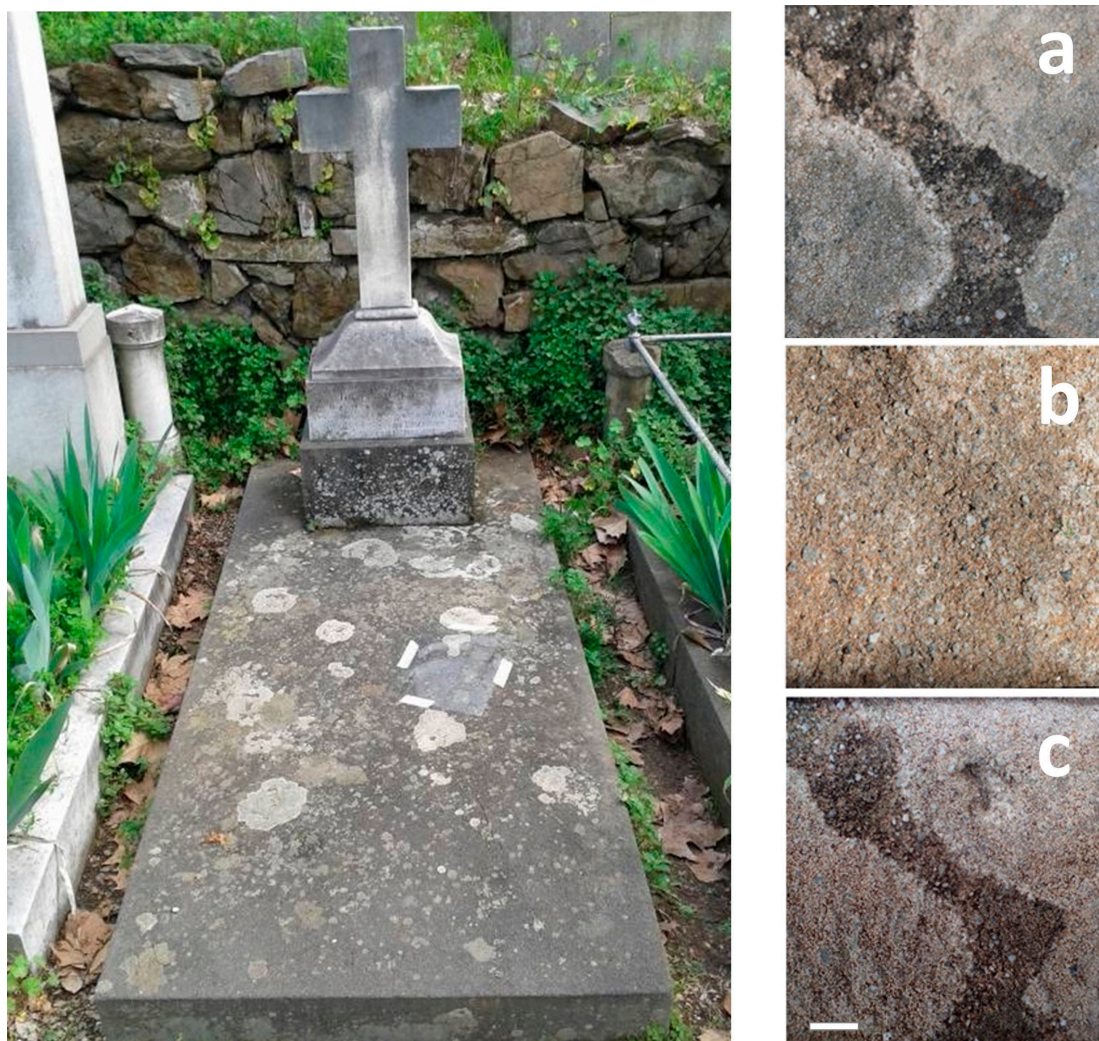
Figure 4. A marble tombstone of the monumental English Cemetery in Florence (Italy). Close-up of an area with the lichen Circinaria caesiocinerea (a). The same area, three months after the lichen's removal by using a soft scraper and deionized water (b). The same area, four and a half years after the mechanical treatment (c). The picture clearly shows that it was unsuccessful as the lichen regrowth pattern is identical to that before the treatment. Bar = 1 cm.
