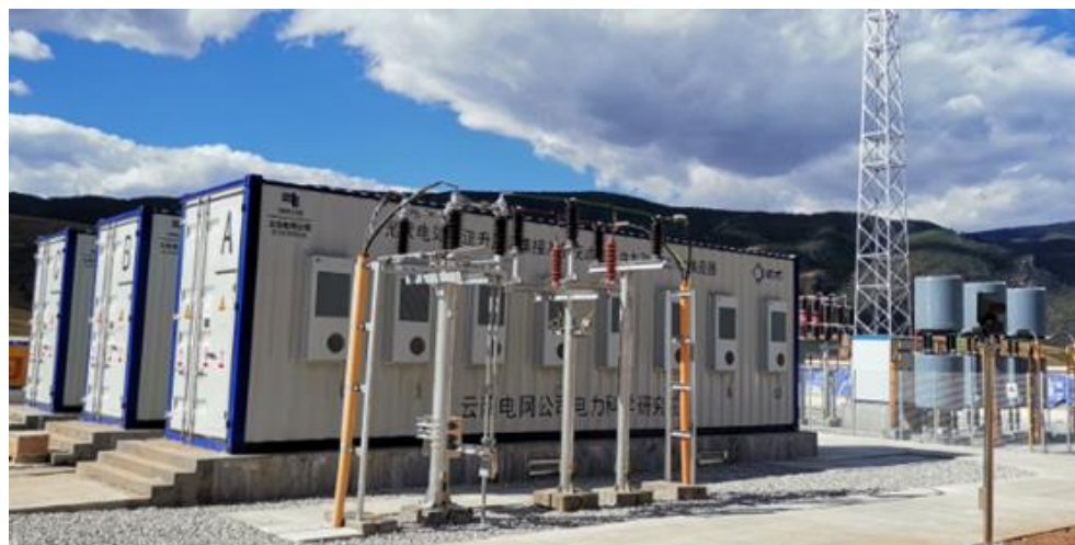
Figure 26. \pm 30 kV MMC converter to simulate HVDC grid.
