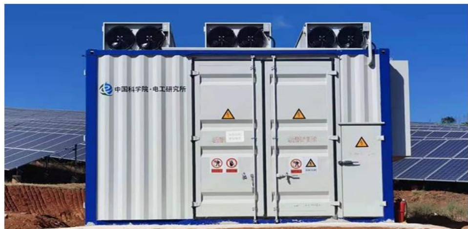
Figure 24. \pm 30 kV/1 MW DC/DC converter engineering prototype.
