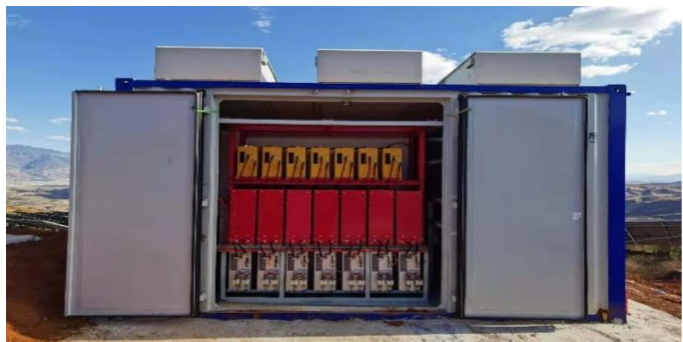
Figure 25. The inside of the \pm 30 kV/1 MW DC/DC converter engineering prototype.
