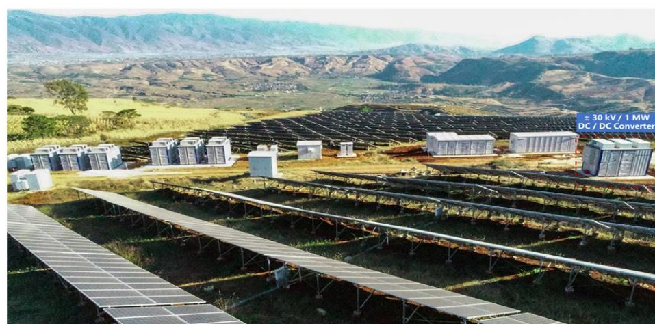
Figure 27. \pm 30 kV/1 MW PV HVDC collection and grid-connection demonstration system.
