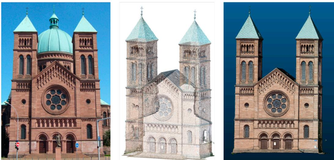
**Figure 2.** The main façade (left), cleaned point clouds (middle), and mesh geometry (right) of the St-Pierre-le-Jeune Church in Strasbourg, France, built from typical Alsatian red sandstone.
