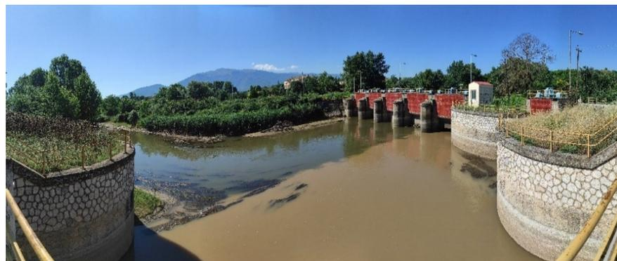
**Figure 3.** A photo of the studied reach. It is the confluence of Aggitis River with Agia Barbara stream and Xiropotamos stream. The different color of the river’s water was due to the different rainfall events in the sub-watersheds. The dam with its movable gates is also depicted on the right of the picture.
