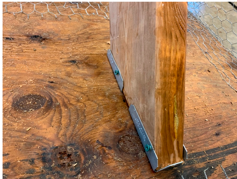
Figure 10. Diagonal connecting to the post and the basket's plywood.
