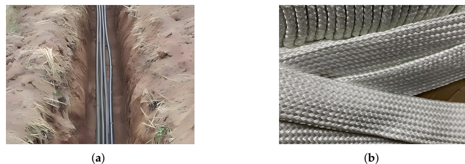
Figure 5. Common embedded fiber placement methods: (a) Directly buried fiber optics. (b) Embedded fiber optic fabrics.
