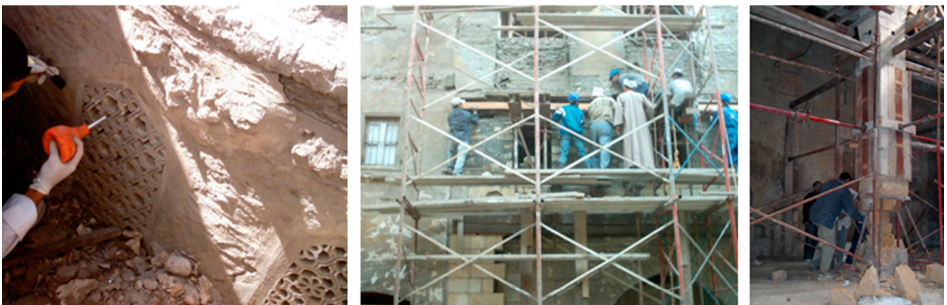
Figure 3. Restoration works on the Dome of Aidkeen Al-Bendqdari in 2006.
