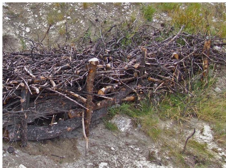
Figure 4. An example—detail of a hillslope log debris dam (bottom). Retrieved from Badía et al. [45].
