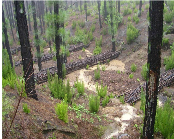
Figure 3. During the application of channel works, re-sprouting of local small trees ( pinus canariensis ), and series of mixed check dams. Retrieved from Lovreglio et al. [43].
